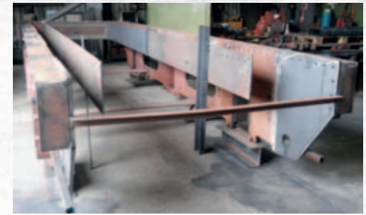
▲ Tender Frames showing new section of Main Frames ready to be welded in position. Also note the new Inner Frames. PHOTO: KEVIN WEST
