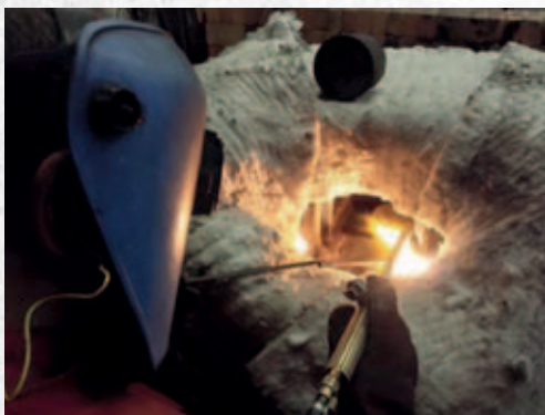
▲ Cast iron welding. PHOTO: OAKWOOD VISUALS
