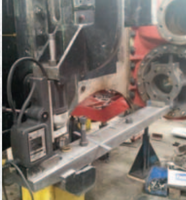
Right Hand Motion Bracket with Bottom Slide Bar in place being drilled.
