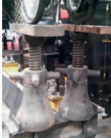
L&NWR Loco Dept jack being used to position the Right Hand Motion Girder.
