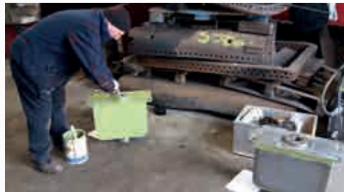
The Trailing Sandboxes being painted in primer at Llangollen.
