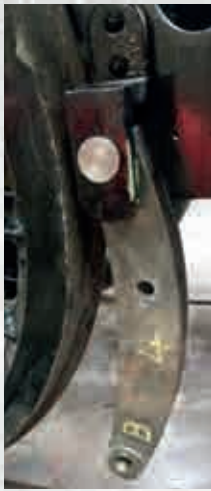
Left: One of the Brake Hangers installed.
