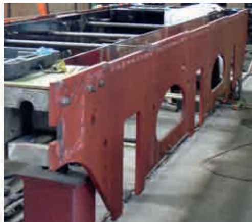
Closer view showing the Main Frame plate drilled and in position.
