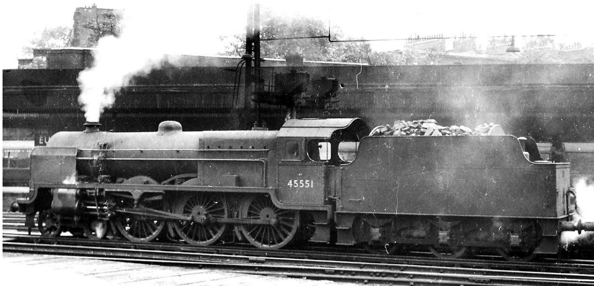
The original 45551 – the last 'Patriot' built. Seen at London Euston platform 7. Note that this loco was fitted with a Fowler high sided tender which gave extra coal capacity. Photo by Martin Welch.
