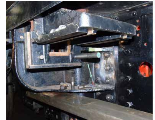
Outside Crosshead Bracket in position.
