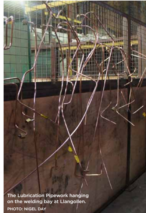
Lubrication Pipework underway on the chassis. PHOTO: NIGEL DAY
