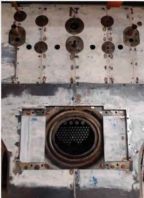
Boiler backhead showing cladding sheets.
