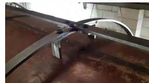
Above: A selection of views of the Crinolines fitted to the boiler barrel and firebox. Photos: HBSS and Kevin West
