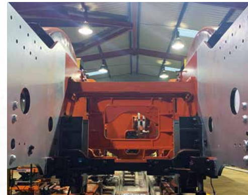
View inside the frames where the firebox will fit.
