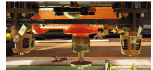
Cylinder Relief Valves, Drain Cocks and Operating Gear trial-fitted to the Left Hand Outside Cylinder. West Shed, 4th February 2020.
