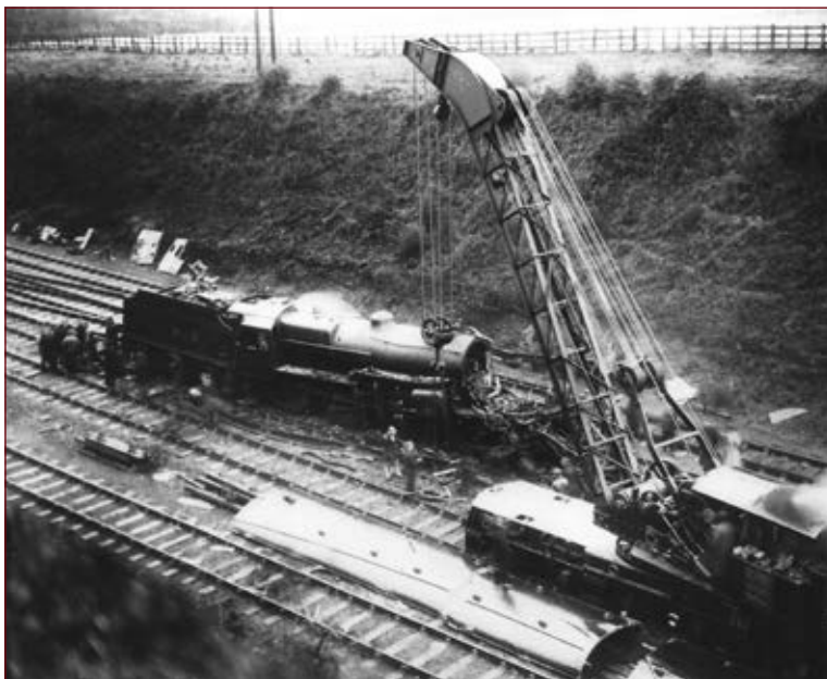
3RD NOVEMBER 1931 • Due possibly to appalling weather conditions, a freight train ran into a train of empty coaching stock just north of Tring station. LMS 2-6-0 Crab No. 13153, hauling a freight train, had been built the previous year. The also then nearly new Craven Bros. 36-ton steam breakdown crane, probably from Rugby, is seen here during the clearing up operation. PHOTO: HERBERT MORRIS, AUTHOR'S COLLECTION
